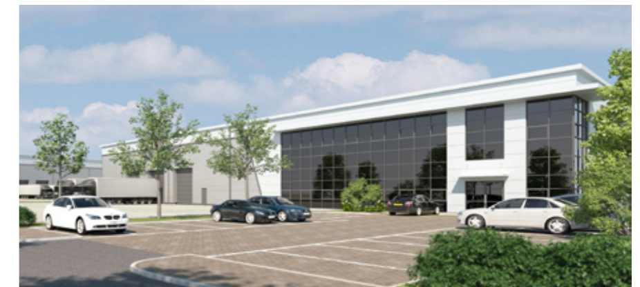
» Low pitch roof cannot be seen from ground level
