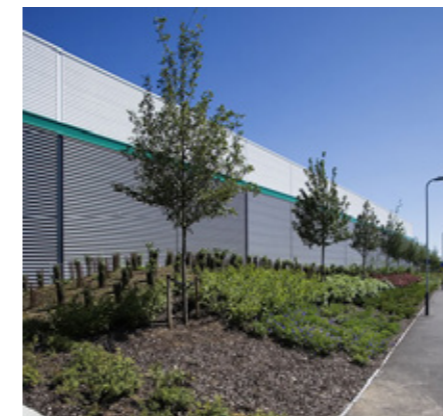
» Pitched roof concealed behind a parapet
